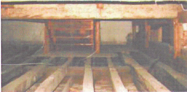
Under Floor Void
