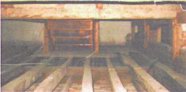
Under Floor Void
