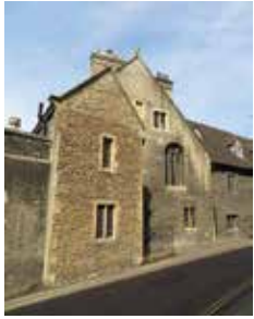
19. The east end of the south range seen from Free School Lane. The pointed arch window used to light a hall in the Master's Lodge. The modern wall on the left is similar in colour and construction to the original Old Court walls
