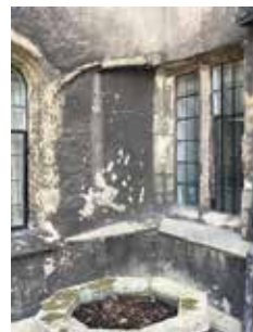
5. The blind half-arch was constructed to avoid blocking a window formed 25 years earlier in the first phase of construction
