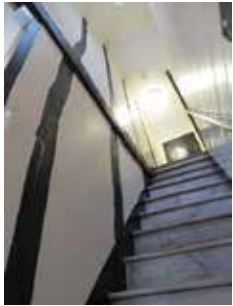
12. Half-timbered partition studs and middle rail on N staircase
