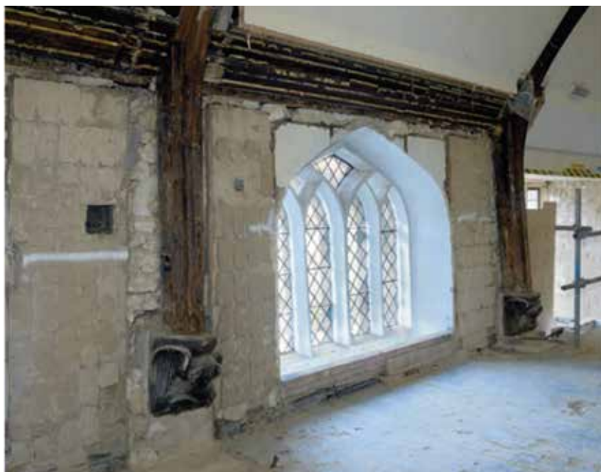
26. Part view of mezzanine floor following the stripping out of the 1949 kitchen. The two corbels supporting the roof trusses had been enclosed in 1981. Photo by Cambridge Archaeological Unit
