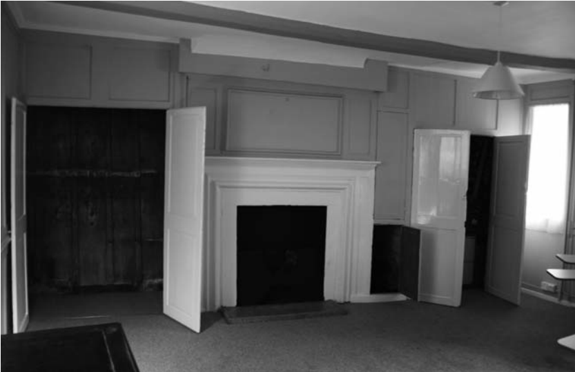
Room Q 1 in Old Court, with features of the 14th century (eg the ceiling beam) and additions and alterations from every century since (eg the 16th century pine panelling inside the cupboard) [Photo: S Laing]
